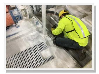
CPE chipped away built up concrete and filled large cracks and holes. All surfaces to be coated were ground to create a proper profile for best product adhesion.
